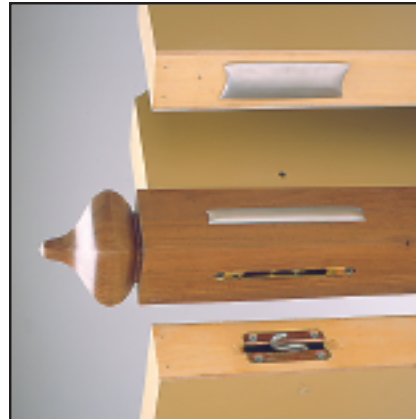
Fig. 1 TYPICAL OFFICE OR EXHIBIT PANELLING WHEREIN THICKER MEMBERS ARE JOINED TO THIN RECEIVERS AT 'T' S & CORNERS
