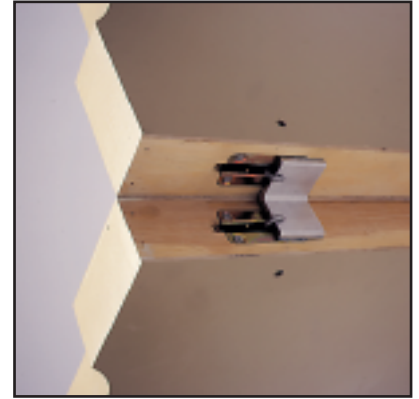
Fig. 3 An Angle Receiver used here with Type 3 Latches provides an inexpensive and simple means of joining panels
