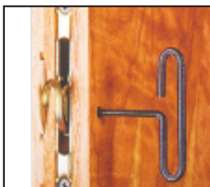
7. Tables and Wall Sections. Type 2 Latch Mortised in Place (see TDSs 62, 82 & 89).
