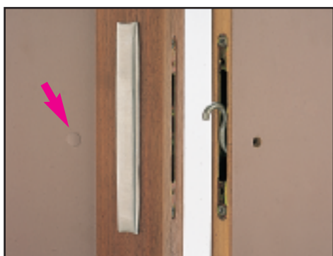
Fig. 2 Typical Prefab Panel Application Where Hole Cover Buttons Are Used (See Arrow) (For information on Large Type 2 Cover Plate Shown, See TDS 128 )
