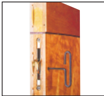
Fig.2 Type 2 Latch mortised in place
