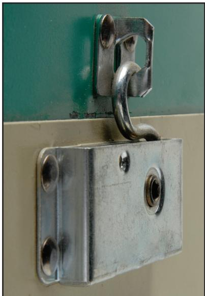
**Fig. 1** In this view the 'OT' Receiver is mounted on the outside of the case and the Type 1 Latch is on the door, with the hinge below. The Latch hook pulling downward on the slanted surface of the Receiver forces the door inward against the case.
